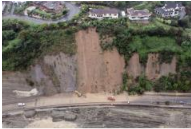
Nelson/Tasman Floods, December 2011. Rocks Road slip. The Nelson Mail.
